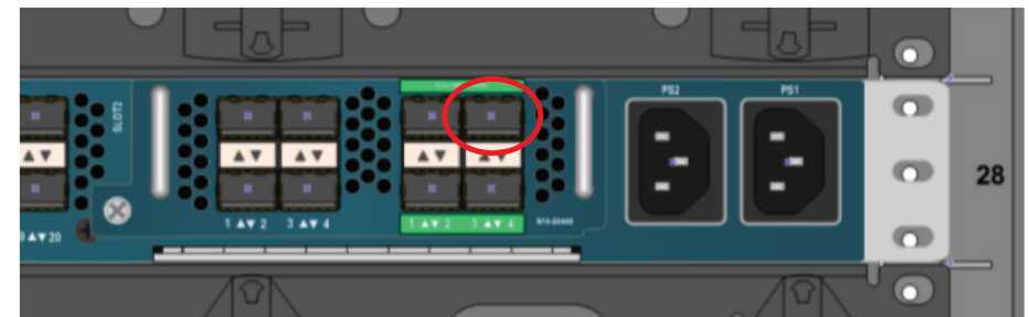
Figure 27 - Uplink port on a Cisco UCS Fabric Interconnect
