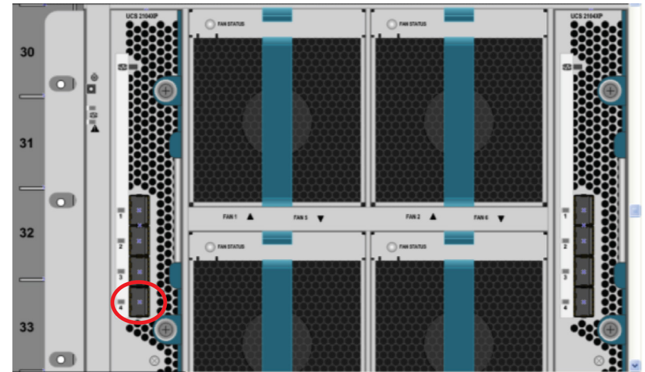
Figure 26 - Identifying a port on a Cisco UCS I/O module
